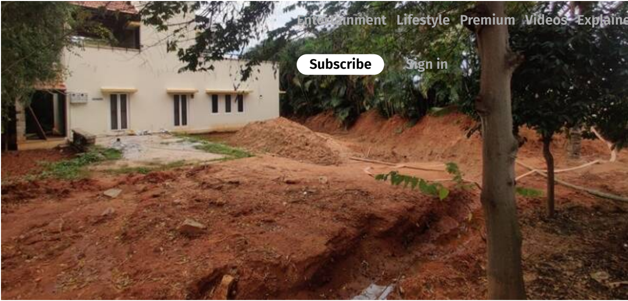
Lake water being pumped out
